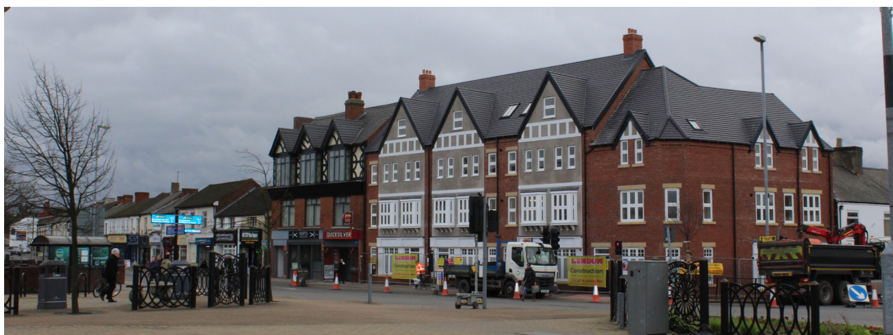
Royal Oak: Formerly the derelict Pick and Shovel pub, £500,000 from NWLDC has helped emh group to develop this site into 14 affordable homes in the centre of Coalville.
